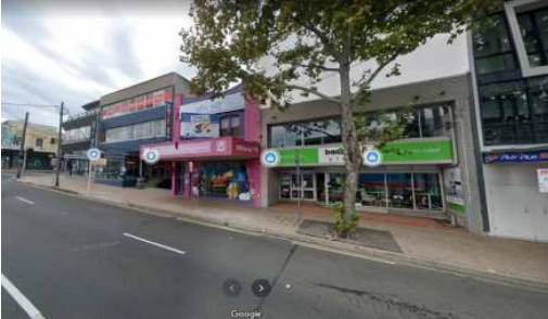
View of: North eastern frontage of the four commercial buildings along Pacific Hwy.
