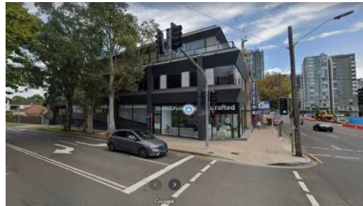
View of: South eastern side of the site from the corner of Pacific Hwy and Hume Street.
